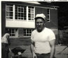
1951 - Carl working on the drive of the church on Eastern Parkway in Louisville.
