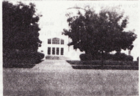
The new 1st Ward Meeting House where I nailed plaster lath on the walls.
